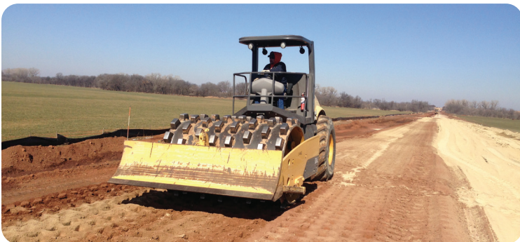
Fly ash being used in road construction project.
